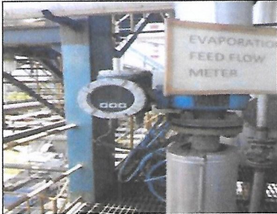
Evaporation feed flow meter
